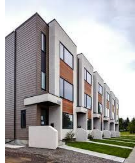
Residential Apartment Complex
